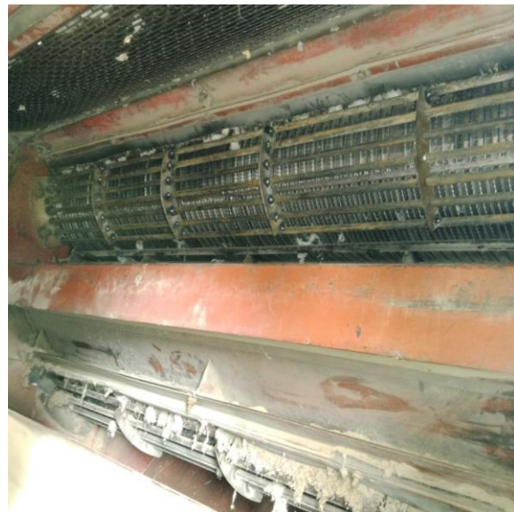
Figure 2. General View of the Section for Cleaning Large Impurities in the UHK Unit, Where the Improved Grating Bar Structure Is Installed, at the "Textile Finance Khorezm" LLC Shovot Cotton Cleaning Branch.
