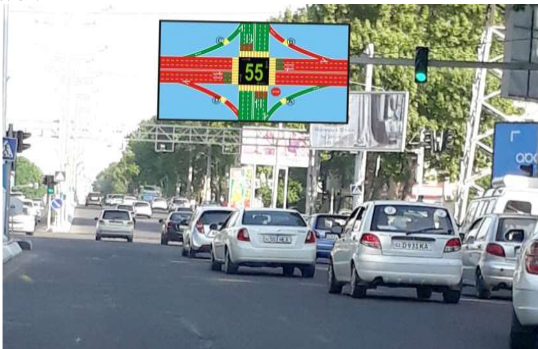
Fig. 4. Installation of a traffic light in front of an intersection.
